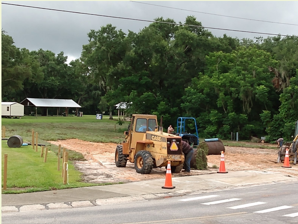
FIGURE 19 PREP WORK FOR SOD
