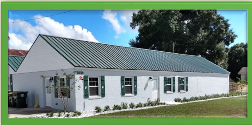
FIGURE 11 25 LAKEVIEW ST COMPLETED PROJECT
