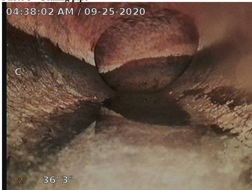
Photo 3 – Scaling pipe
