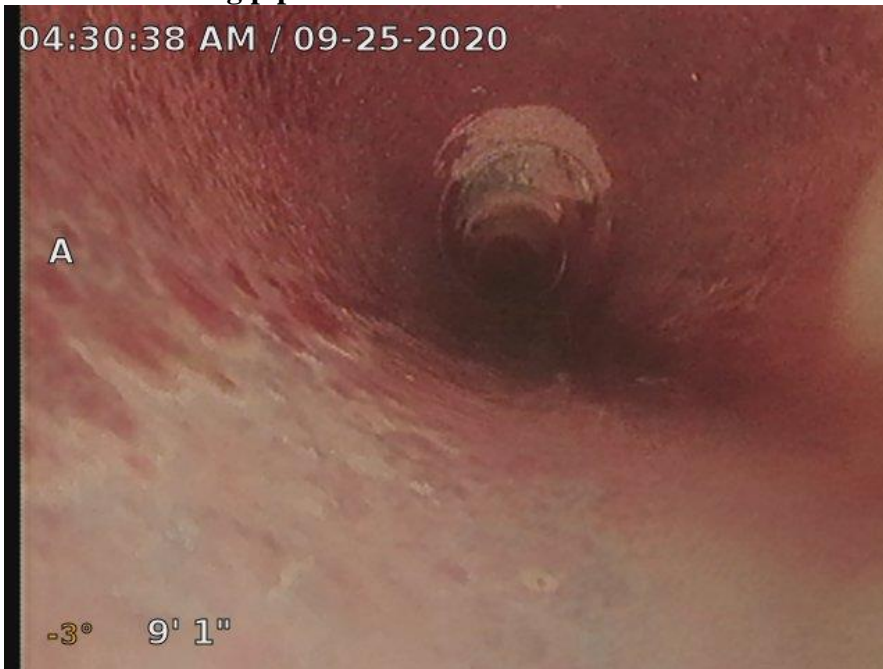
Photo 1 – Scaling pipe
