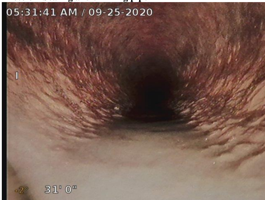
Photo 8 – Scaling and thinning pipe
