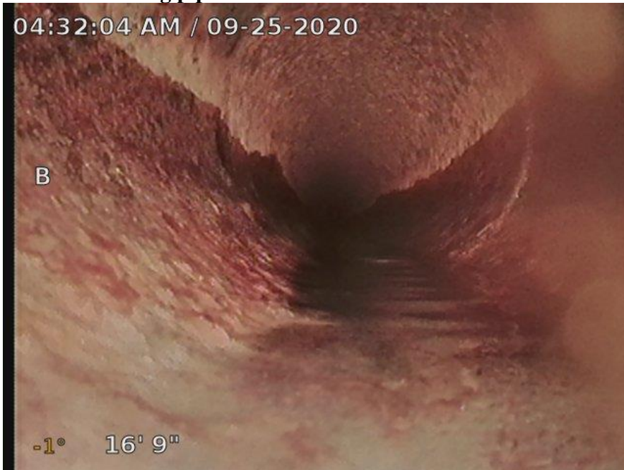
Photo 2 – Scaling pipe
