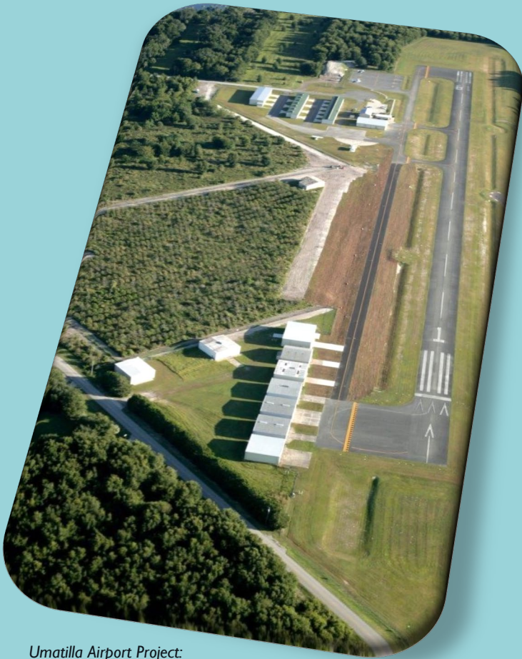
Umatilla Airport Project: Completion of Parallel Taxiway
